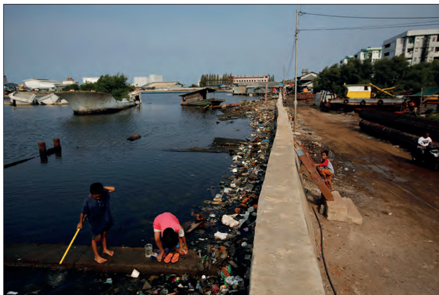
Figure 5 – The current sea wall at Jakarta
